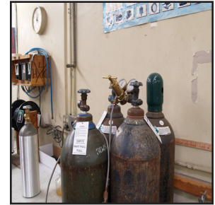
Fig. 35 Large compressed gas supply bottle
