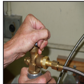
Fig. 38e Shut off supply valve of small bottle
