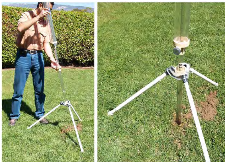
Fig. 24. Left: lowering GP into Tripod and Borehole.
